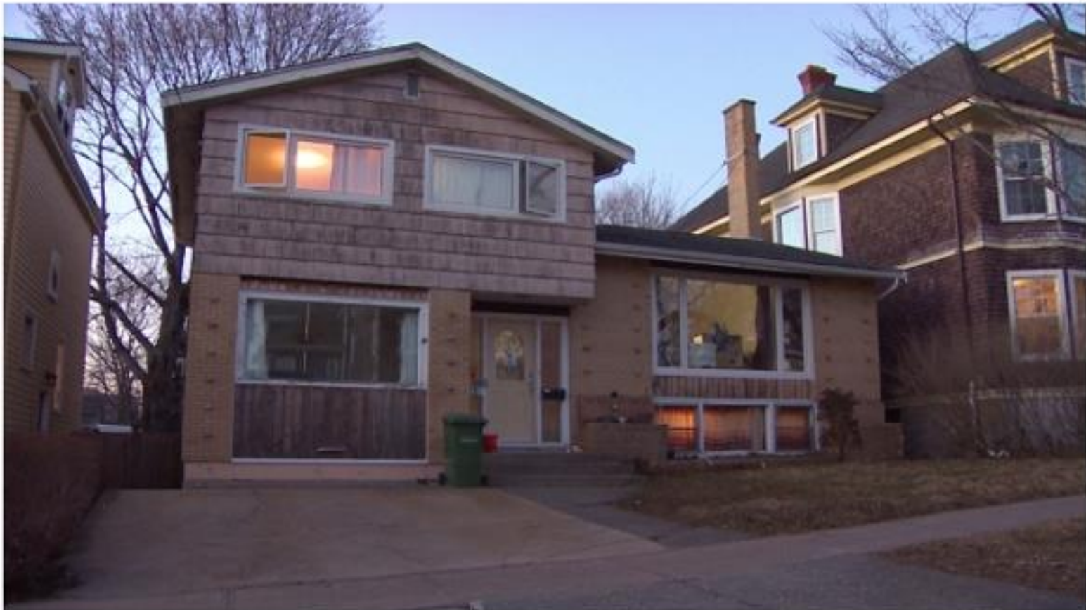
Planning officials are investigating whether this house at 6299 Payzant St. in Halifax complies with land-use bylaws. (CBC)
