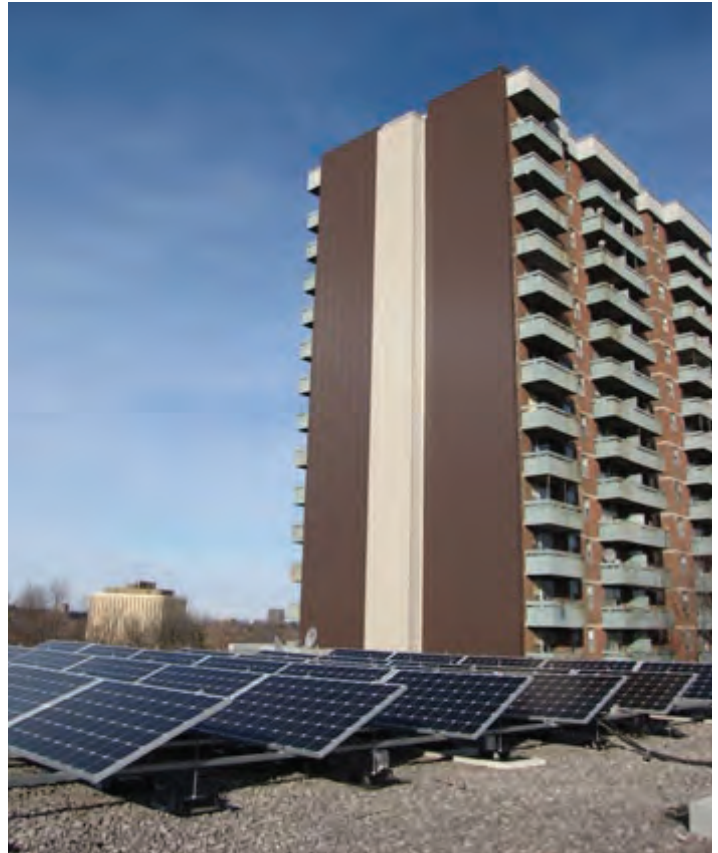
OCH installed an 8,000 square foot solar wall on one of their high-rise buildings, reducing natural gas consumption by 21 percent.
