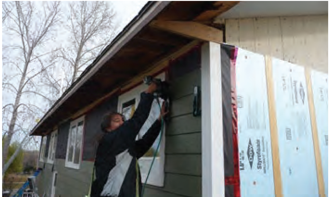
BEEP crew siding housing after insulating exterior walls, helping to reduce energy consumption and costs to low-income homeowners.
